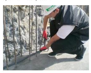
In comparison to plastic or resin based swellable tapes, which do not alter their structure during swelling, KÖSTER Quellband 2520 breaks down during the swelling process and the resulting paste seals all cracks and voids permenantly.
