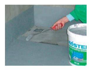
**Surface Preparation** - Surfaces shall not be below 5 °C and must be clean, dry, structurally sound and free of efflorescence, grease, oil, form release agents and curing compounds. On painted surfaces, remove all blistered or peeling paint to a sound substrate. Remove all gloss by sanding.
