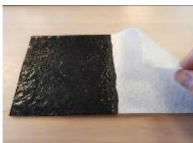
**Subsequent Layers** - Apply at least 2 (unthinned) layers (3 layers are better) by brush, roller or airless spray. Wait apr. 24
