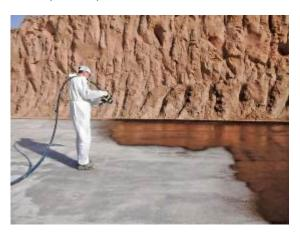
**Subsequent layers** – Stir powder and liquid components thoroughly (for 3 minutes using a motorized mixer 400rpm and suitable mixing paddle) prior to application. The mixed material must be homogeneous and lump free.
