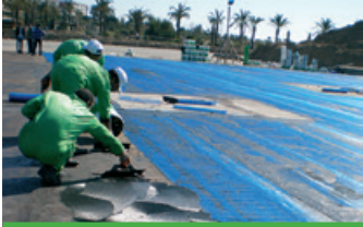
Temel bohçalama Under slab waterproofing
