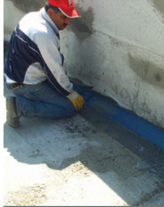
Filling of tie-rod holes and forming of fillets
