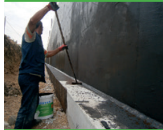
External basement wall
