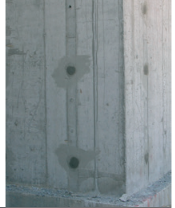
Filling of tie-rod holes and forming of fillets
