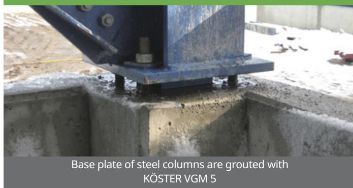
Base plate of steel columns are grouted with
