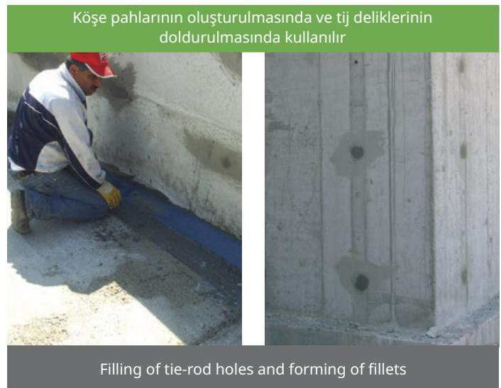
Filling of tie-rod holes and forming of fillets
