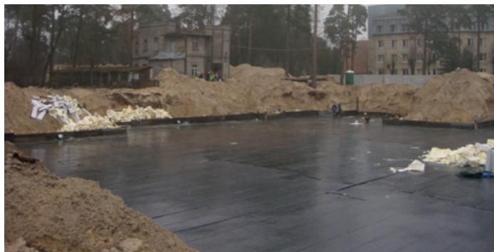
EN KÖSTER KSK SY 15 consists of a highly tear resistant, 2-layer cross laminated polyethylene foil with a plastic bitumen / rubber adhesive and sealing compound. It is cold applied and therefore no hot air or propane gas welding is required for application. Due to its high ductility it can easily be applied to difficult details.
