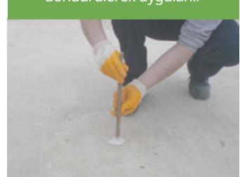
The anchor bolt is inserted into the hole by turning it clockwise
