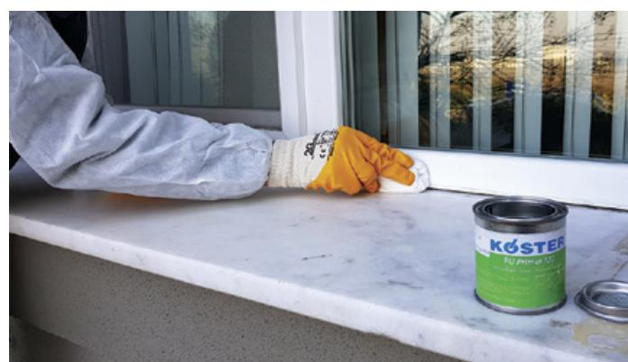
EN KÖSTER PU Primer 120 promotes the adhesion of polyurethane sealants to non-porous surfaces, such as rigid PVC, aluminium, glass and glazed tiles. The primer also cleans the surface from grease and activates the surface.
