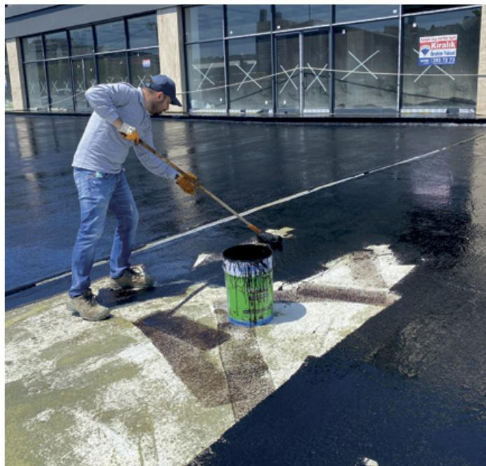
**EN** KÖSTER Bituflex-1K is a one component, bitumen-extended hydrophobic polyurethane waterproofing material with low solvent content.
