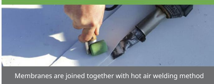
Membranes are joined together with hot air welding method
