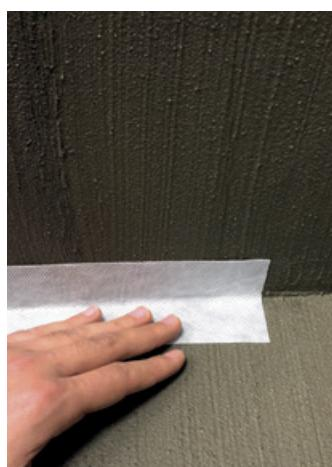
**EN** KÖSTER Fixband-Vlies is a butyl based, self adhesive joint sealing tape with fleece-laminated upper side and is used for the secure bridging of joints, wall floor junctions and in areas prone to cracking. The fleece laminated upper layer of the material has good adhesion to cement renders and mortars. In wet room waterproofing applications it is used in combination with KÖSTER BD 50.
