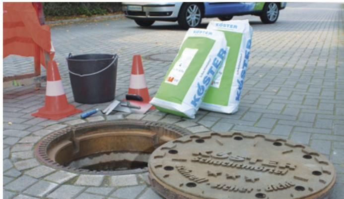
**EN** KÖSTER Grout S 50 is a cement based, flowable consistency, shrinkage compensated grout. The material is one component and is easily prepared by mixing with fresh water only. KÖSTER Grout S 50 is fast setting and develops early strength. The cured material has high final compressive strength. KÖSTER Grout S50 is normally used for raising manhole covers, installing traffic signs and flag poles, repairing cavities in concrete floors, concrete anchorages and similar applications.
