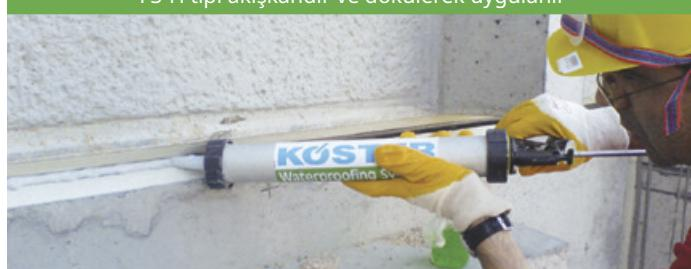
FS-V type is in paste form and is applied with a mastic-gun,
