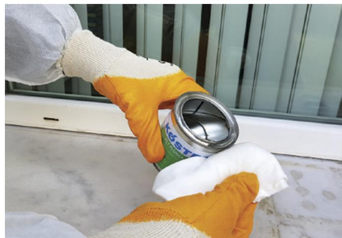
EN KÖSTER PU Primer 110 promotes the adhesion of polyurethane sealants to porous surfaces, such as concrete, cement, wood and teak etc. The primer penetrates the material and eliminates residual dust.
