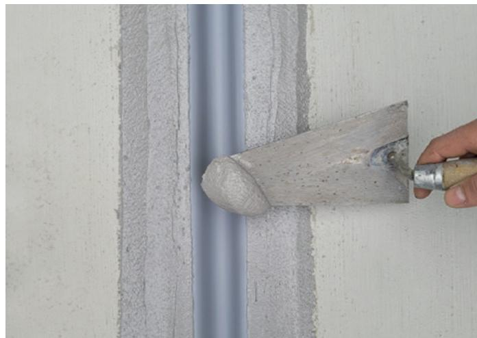
**EN** KÖSTER KB Fix is a two-part, epoxy based, high performance adhesive and repair mortar. The material is thixotropic and in paste form, contains no solvents. The material has high adhesion strength to concrete, mortar, metal, wood and many other building materials without the use of a primer. The cured layer is waterproof and has high compressive strength. Horizontal, vertical or overhead applications are possible.
