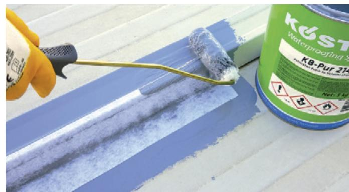
**EN** KÖSTER KB-Pur 214 FLEX is a polyurethane based waterproofing product with 1000% elasticity. It is single component, cures rapidly to form a seamless and elastic waterproofing layer. It is easily applied with a brush, roller and airless gun. It provides an economical and long-lasting solution in the most difficult waterproofing details.
