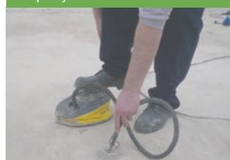
The holes are cleaned from dust and loose particles with compressed air and a brush
