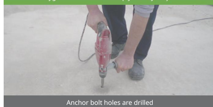
Anchor bolt holes are drilled
