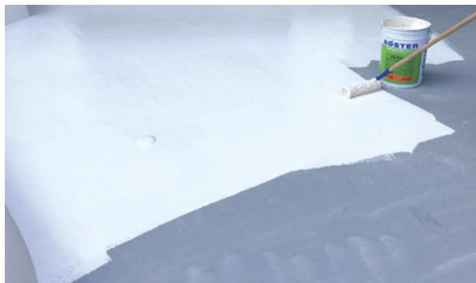
**EN** KÖSTER KB-Pur 2K-Topcoat SW is a two component and fully aliphatic polyurethane based top-coat. Once cured it produces a very tough and chemically resistant protection layer, which is also UV resistant. Service temperature is -40°C to +80°C and outdoor stability is perfect.
