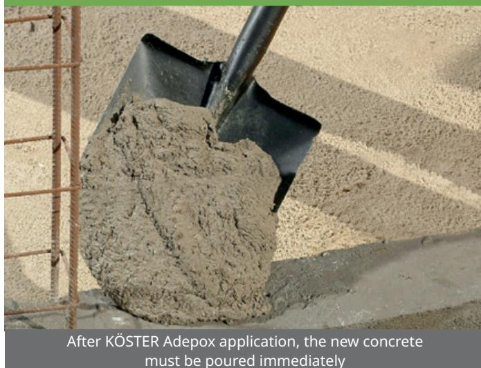
After KÖSTER Adepoxy application, the new concrete must be poured immediately
