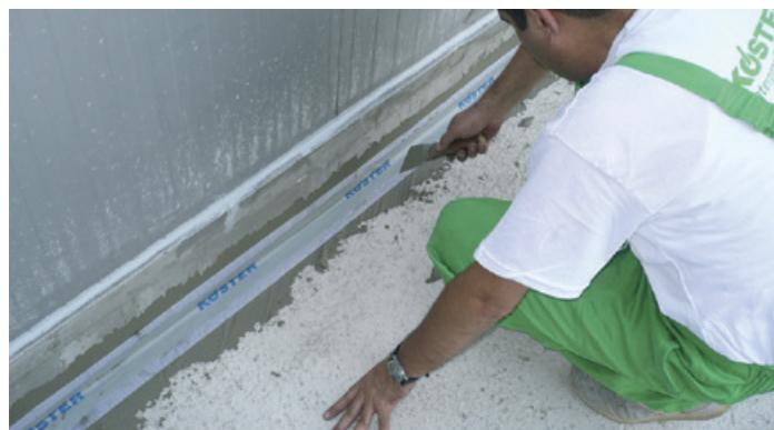
EN KÖSTER K120-W Sealing Tape is a highly flexible joint sealing tape made of high quality elastomeric material, with a PP non-woven fabric laminated on both sides. It is compatible with many liquid waterproofing materials, including cement based slurries.
