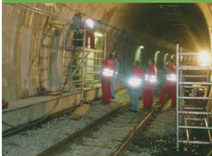
Application of epoxy injection resin
