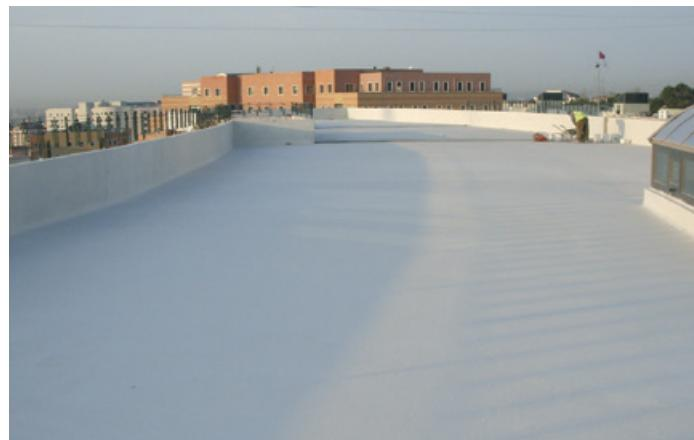
**EN** KÖSTER NB Super Elastic WHITE sealing slurry is a highly flexible and UV-stable waterproofing coating with excellent application properties. The finished layer is white colored and reflects the radiation heat.
