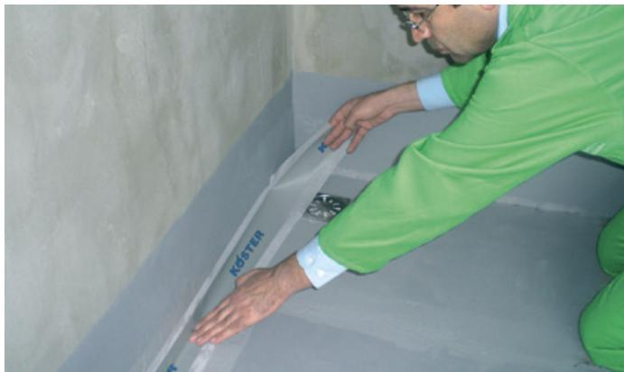
**EN** KÖSTER K120 is a elastic joint sealing tape for the safe connection of crack prone areas. The tape consists of an extruded elastomeric center part, which is highly flexible and waterproof. On both sides a fine-textured mesh is laminated into this elastomeric tape, which secures a strong and permanent bond with the liquid applied waterproofing layers.
