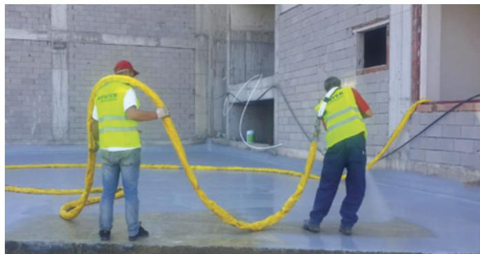
**EN** KÖSTER KB-Pur 570 is a pure polyurea waterproofing product, which consists of 2 components and is applied with special high pressure hot spray equipment.
