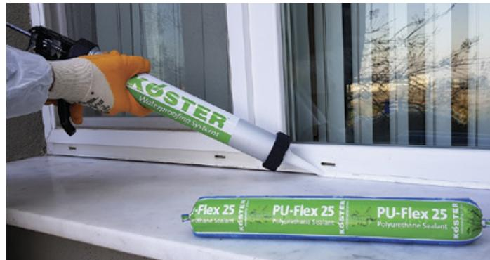
EN KÖSTER PU Flex-25 is a highly elastic, low modulus polyurethane sealant, with good UV resistance and excellent adhesion to typical construction materials.
