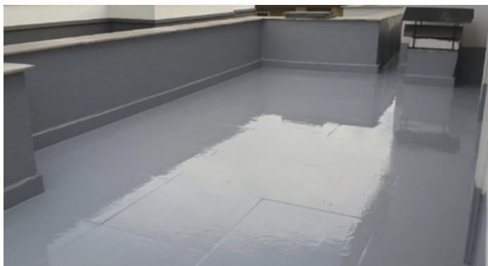
**EN** KÖSTER KB-Pur 214 is a one part, polyurethane based, liquid applied waterproofing material. After application the material cures with air moisture to form a seamless, elastic, crack bridging and walkable membrane. The cured membrane has high adhesion strength to concrete, masonry, plaster, mortar and many similar building products.
