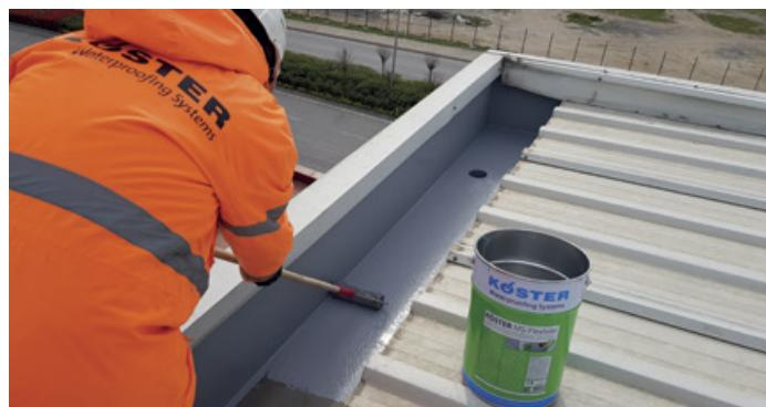
**EN** KÖSTER MS-Flexfolie is a premium quality, liquid applied waterproofing product based on MS-Polymer technology. KÖSTER MS-Flexfolie is solvent free and does not contain isocyanates. The material cures to form a very elastic (500%), crack bridging and impermeable waterproofing layer.
