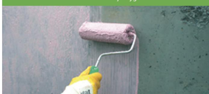
High adhesion between concrete and cement render
