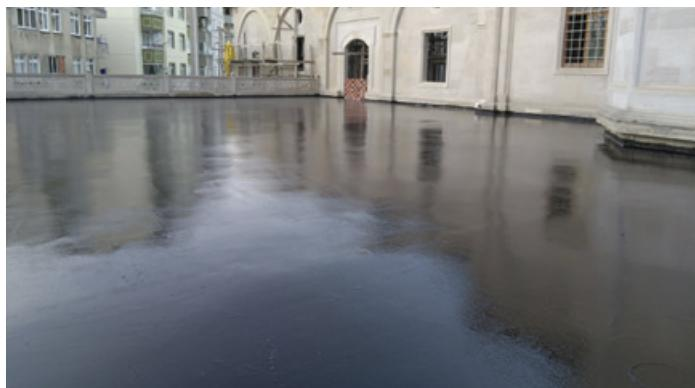
EN KÖSTER KB-Pur 223 is Bitumen-PUR based, two component waterproofing product with very high elasticity % 1500 and good adhesion to many different substrates. The mixed components are applied with a roller, brush or airless spray. The cured membrane is of black color and has a service temperature of -30°C to +80°C.
