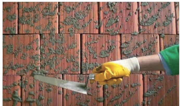
**EN** KÖSTER Latex emulsion is a water based, plasticizer free, dispersion based synthetic rubber compound. KÖSTER Latex emulsion is compatible with all standard cements, mortars and cement based adhesives.
