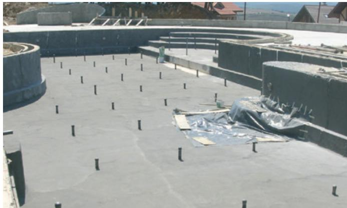
EN KÖSTER NB Elastic 2K sealing slurry is a two component mineral coating with excellent elastic properties. It can be applied on concrete and masonry surfaces which are in danger of cracking. KÖSTER NB Elastic 2K has very good adhesion on mineral based, absorbent and non absorbent substrates.
