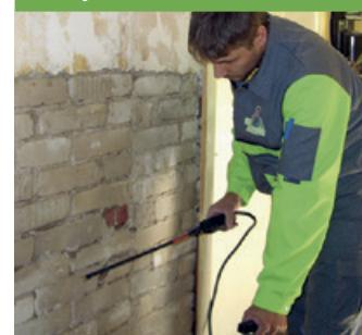
Existing render is removed before application than wall is primed with Polysil TG 500
