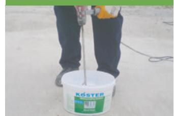
Bond Paste components are mixed with a motorized mixer
