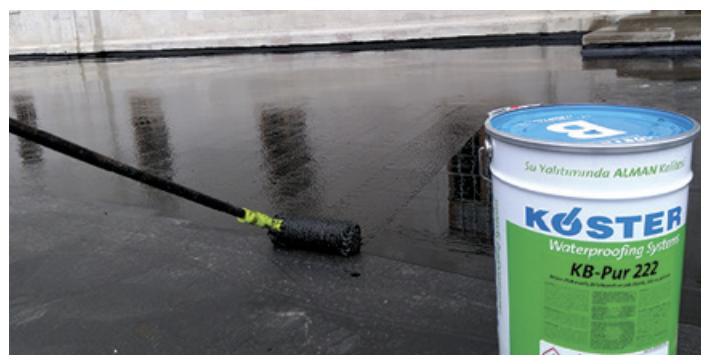
**EN** KÖSTER KB-Pur 222 is bitumen-PUR based, two component waterproofing product with very high elasticity %2000 and good adhesion to many different substrates.
